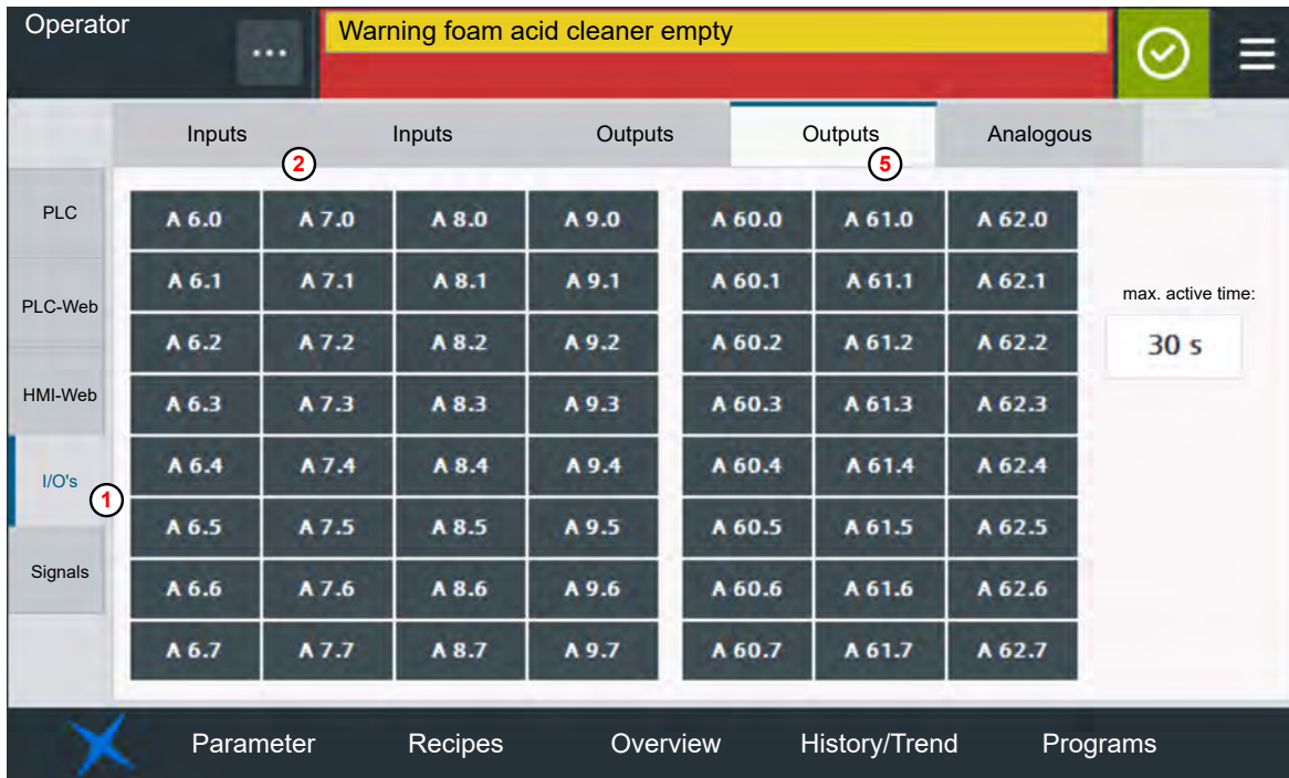
Fig. 76: [Diagnostic] -> [I/O's] -> [Outputs 2]
